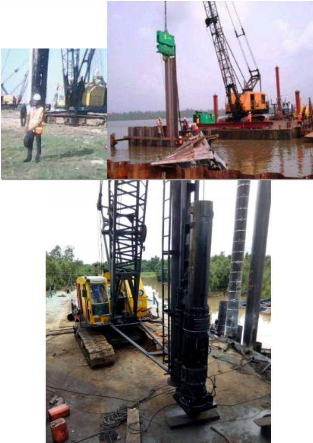
Vibro Installation of Steel Sheet Piles and Impact Hammer Installation of Steel Casings at Delta State
