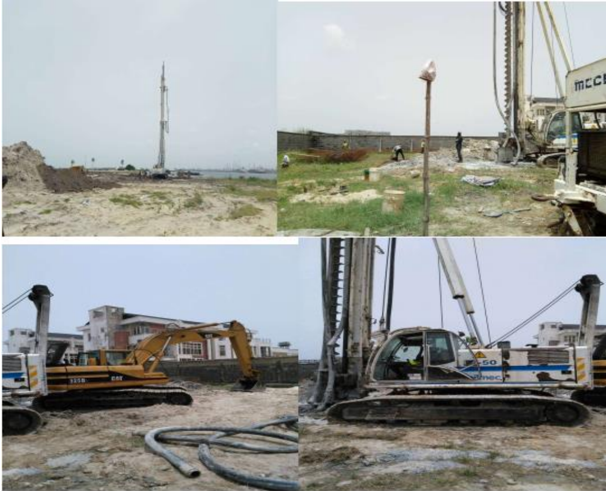
CFA Bore Piling and Precasting Piling Works, Lekki, Lagos
